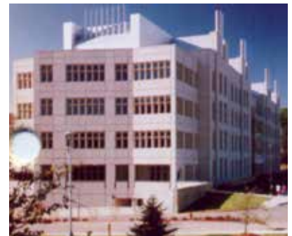
Figure 8 Use of vertical projections.
