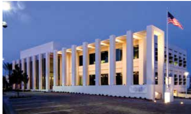
Figure 4 Detached sunshades. (Courtesy © Brian Gassel/TVS & Assoc.)
