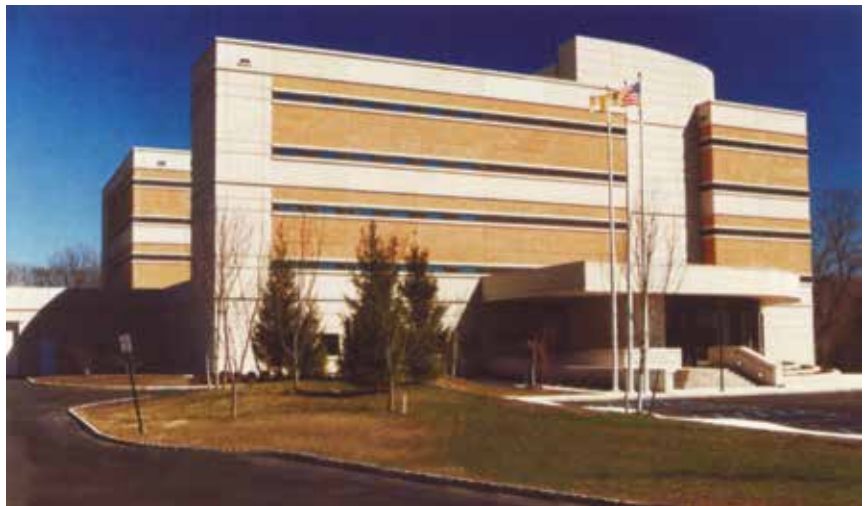
Figure 38 Insulated sandwich wall panels with exposed interior. Morris County Correctional Facility, Morris Township, NJ. Hellmuth, Obata & Kassabaum.
