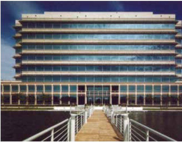
Figure 2 Horizontal sunshade. (Courtesy © Brian Gassel/TVS & Assoc.)
