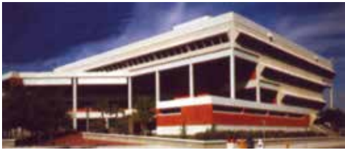
Figure 13 Hooded shading device.
