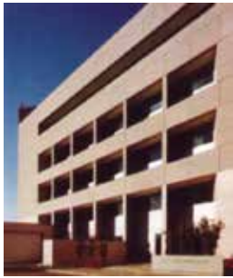
Figure 10 Deep recessed windows. (Courtesy © Glen Allison)
