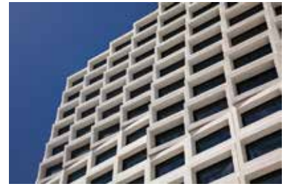
Figure 7 Precast window openings that tilt in multiple directions.
