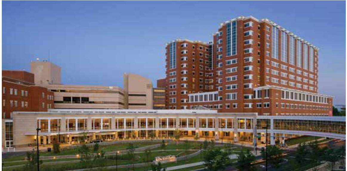
Figure 36 Insulated sandwich wall panels. University of Kentucky Albert B. Chandler Hospital's Pavilion A, Lexington, Ky., GBBN Architects and AECOM, Inc.
