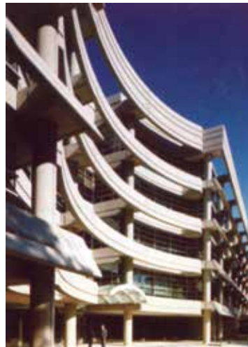
Figure 4 Detached sunshades. (Courtesy © Brian Gassel/TVS & Assoc.)
