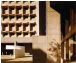
Figure 11 Deep recessed windows and overhang (eggcrate device). (Courtesy © MBA)
