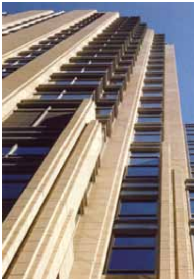
Architectural precast panels articulated in an ashlar pattern clad Northwestern Memorial Hospital in Chicago, Ill.
