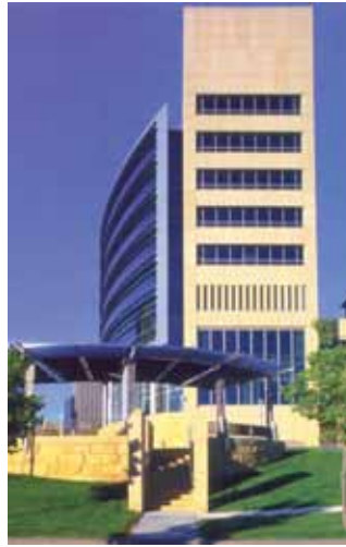
Precast cladding blended with the stone base of the Federal Reserve Bank in Minneapolis, Minn.
