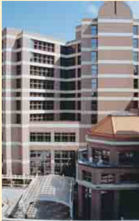
Two colors of precast concrete were used on the M.D. Anderson Cancer Center in Houston, Texas. Recessed window openings on the bed tower provide shadowlines and detail to the overall façades.
