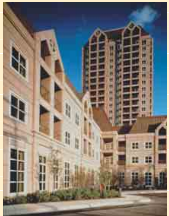
The USAA Retirement Center in San Antonio features precast concrete throughout the façade. Window panels on the low-rise structures highlight a variety of profiles and treatments, as do the balconies and window areas of the tower of the project.
